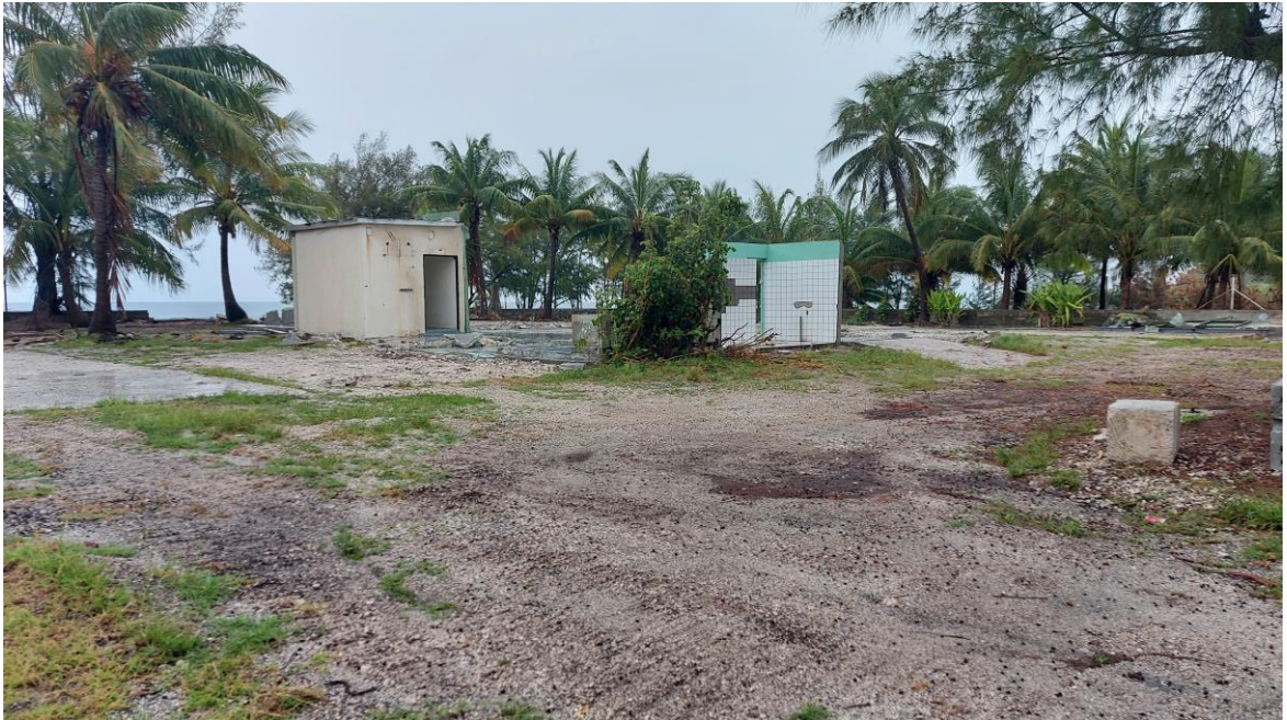
Figure 0 : Dallage et structure hangar
