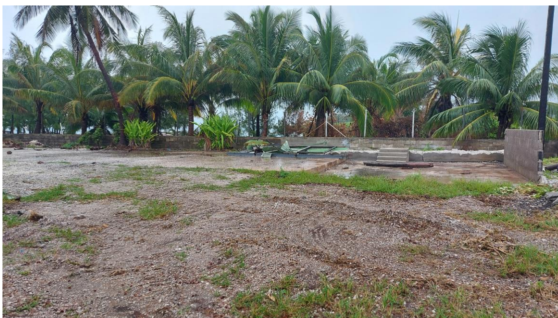
Figure 3: Fondation hangar + auvent
