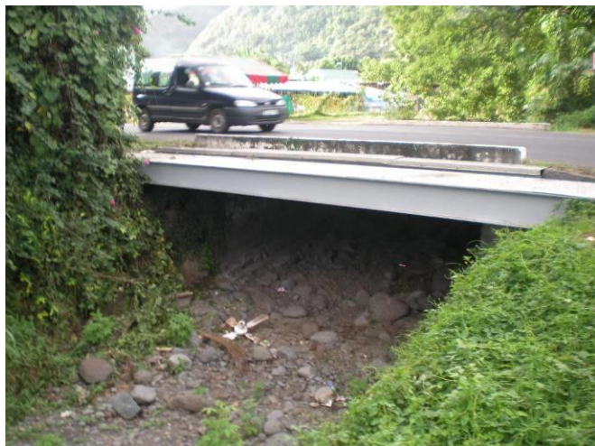
Photo 12: OA franchissement RT (vue aval)
