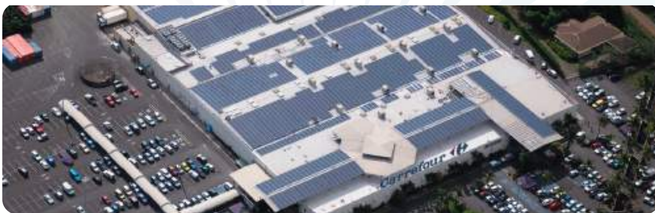
Installation photovoltaïque (© Eco Energy - Carrefour Punaauia)
