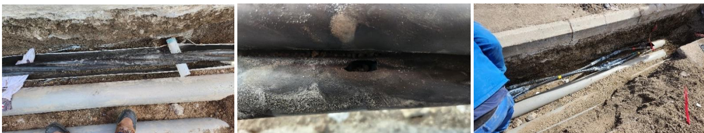
Cable souterrain HTA terminé
