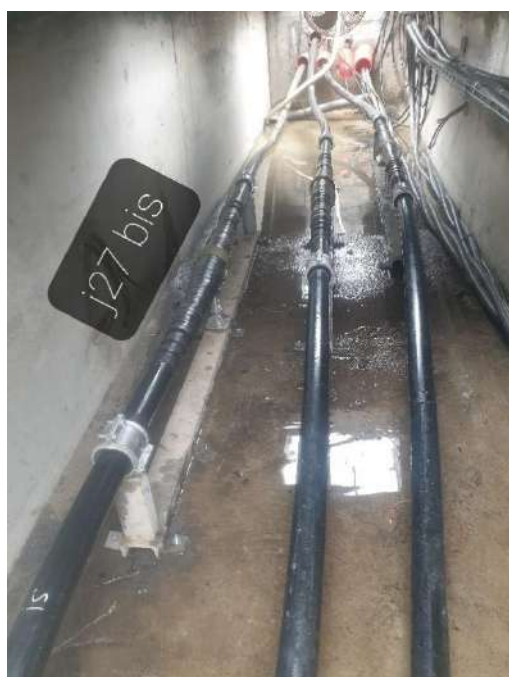
Figure 1 - Jonctions HTB 90kV
